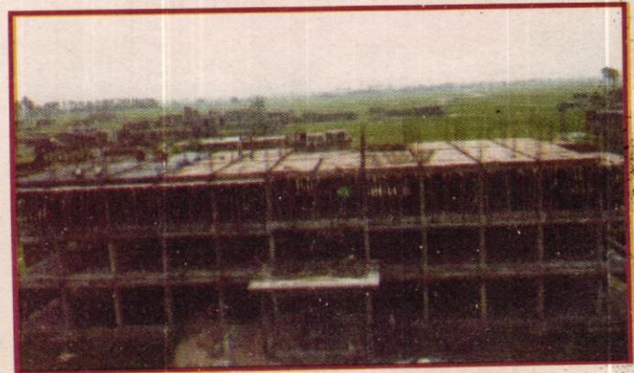
Under construction site of New Building
